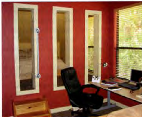
TUCK ME IN: A sleeping "nest" off the home office in Ed Binkley's own Florida residence makes clever use of what would otherwise be an unused cavity in the framing.
